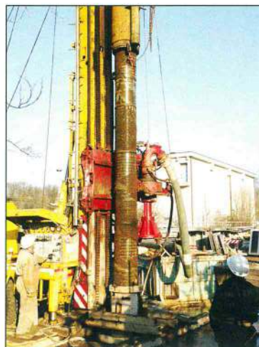
Left column: new 1,200mm-diameter steel casing being installed to 13m depth
