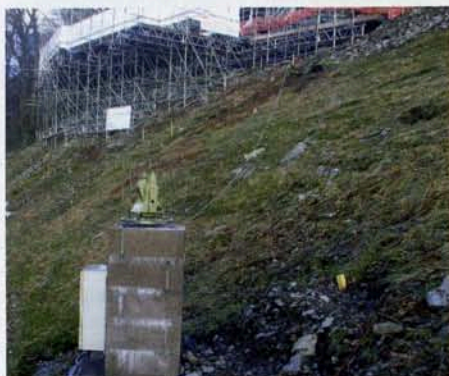
The project required great accuracy in its execution
